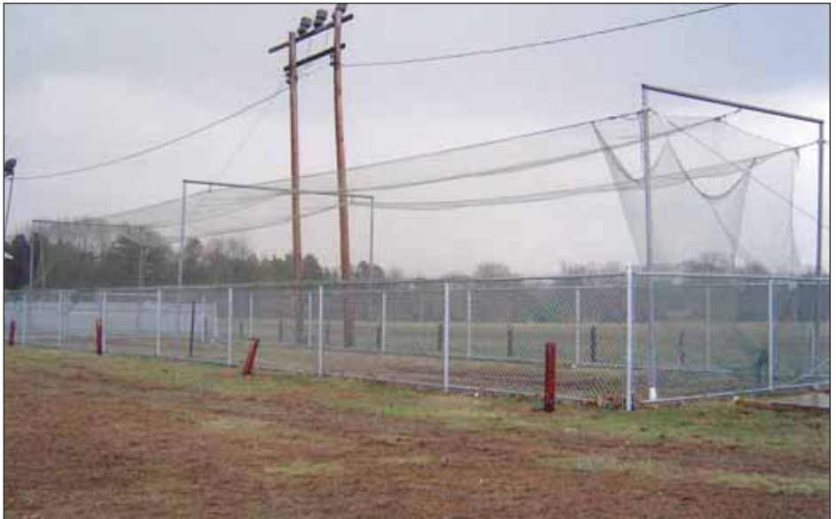
Protect players inside and out of batting cages by installing a second fence or netting around the primary cage. Note posts to keep cars from running into the fence, as well.
